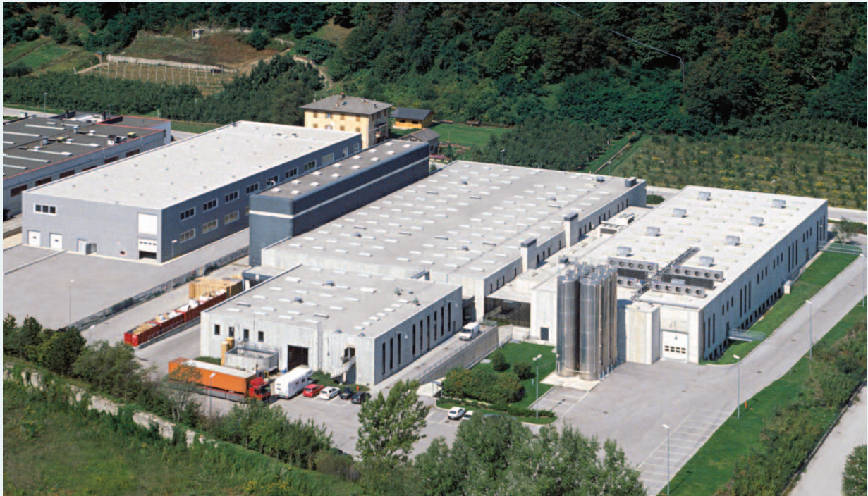
Below, a view of the Coster 3 and Coster 4 plants located in Caldonazzo, Italy. Coster 3, to the right in the photograph, is one of the most advanced and highly automated plants in the aerosol valve sector. Automation is governed by an integrated, computerized system that continuously monitors the entire production flow, from the dosage of the raw materials in the silos to the moulding, collection of moulded components by laser-guided robots, sorting and finally packaging and preparation for shipping. Also manufactured in Coster 3 are the valves used in the Coster 4 facility, dedicated exclusively to the production of Bag-On-Valves. Left, Coster USA, Inc., South Elgin, Illinois: the factory is located near Chicago's O'Hare Airport. Assembly of 1" valves and bag placement are performed at this facility.
